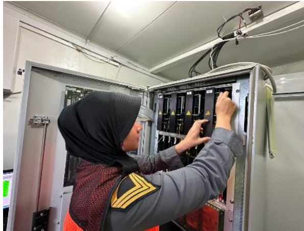
Gambar 21. Pergantian modul MOD/PA CLR
