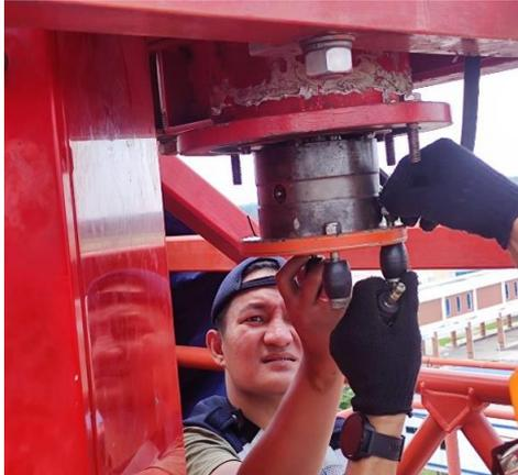
**Gambar 11.** Memasang *Flexible Coupling*
