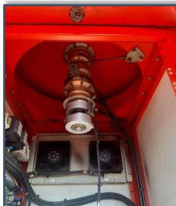
Gambar 4. *Rotary joint*
